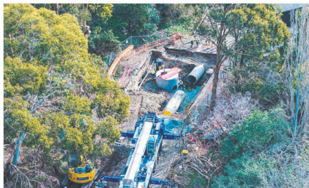
Gross pollutant trap being installed near tip face at McRobies Gully. Designed to limit the flow of litter and pollution into the Hobart Rivulet and protect wildlife.
